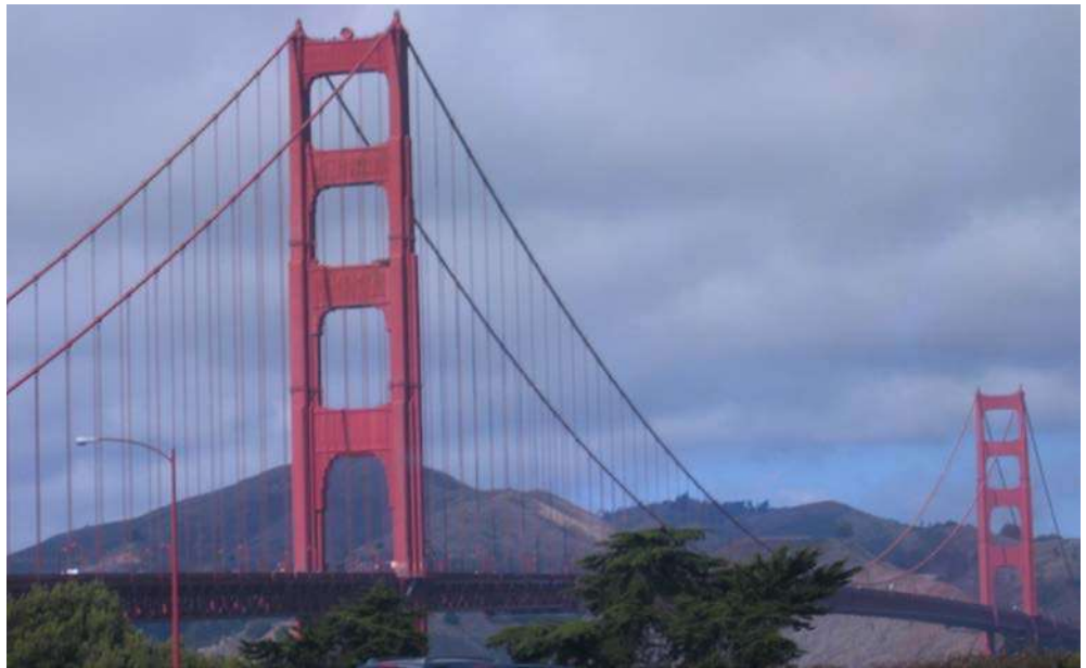
Figure 3.1.19 Cable-Supported Bridge: Suspension Cables and Hangers
