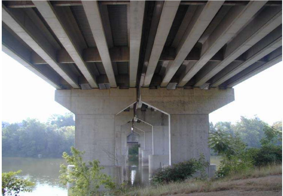
Figure 3.1.79 Cantilever or Hammerhead Pier
