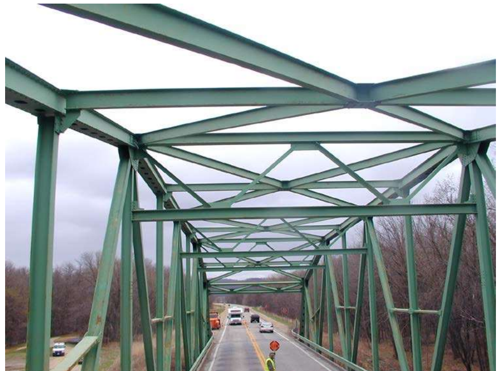
Figure 3.1.67 Top Lateral Bracing and Sway Bracing
