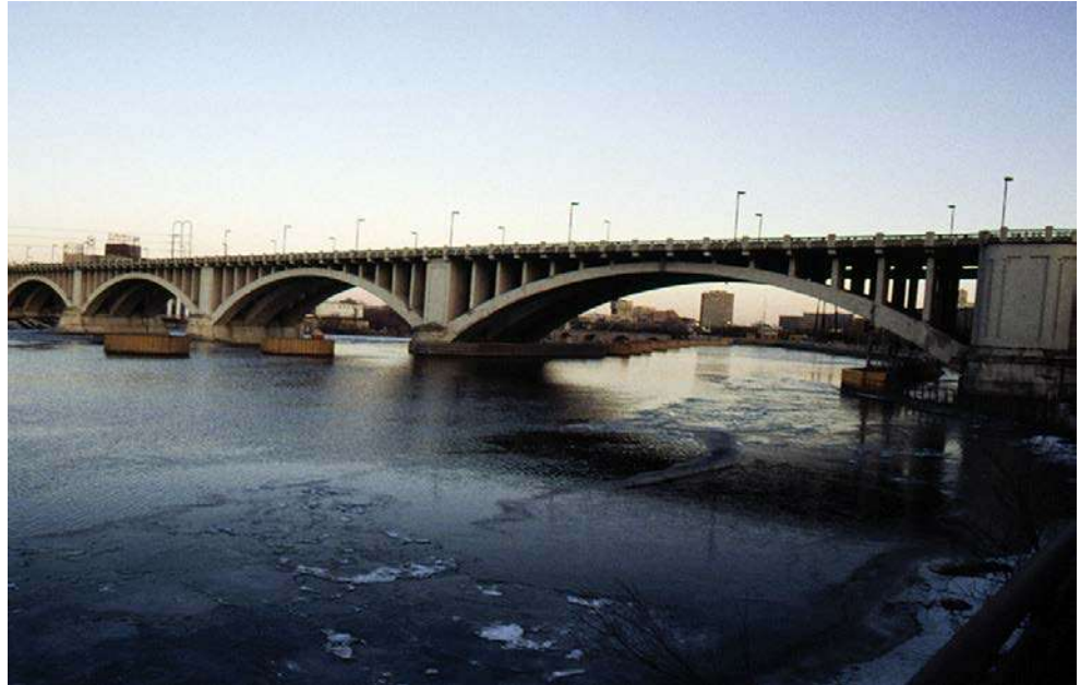
Figure 3.1.54 Deck Arch Bridge
