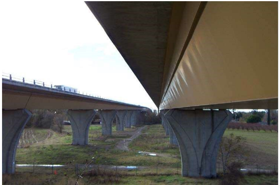
Figure 3.1.51 Box Girder Bridge
