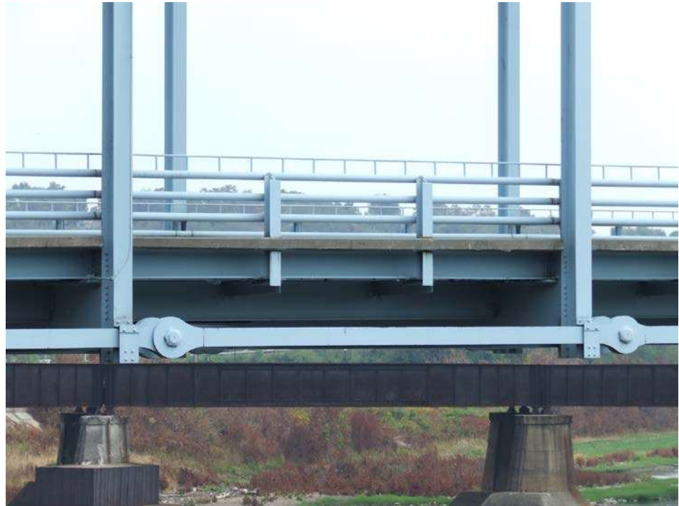
Figure 3.1.22 Pin-Connected Eyebars
