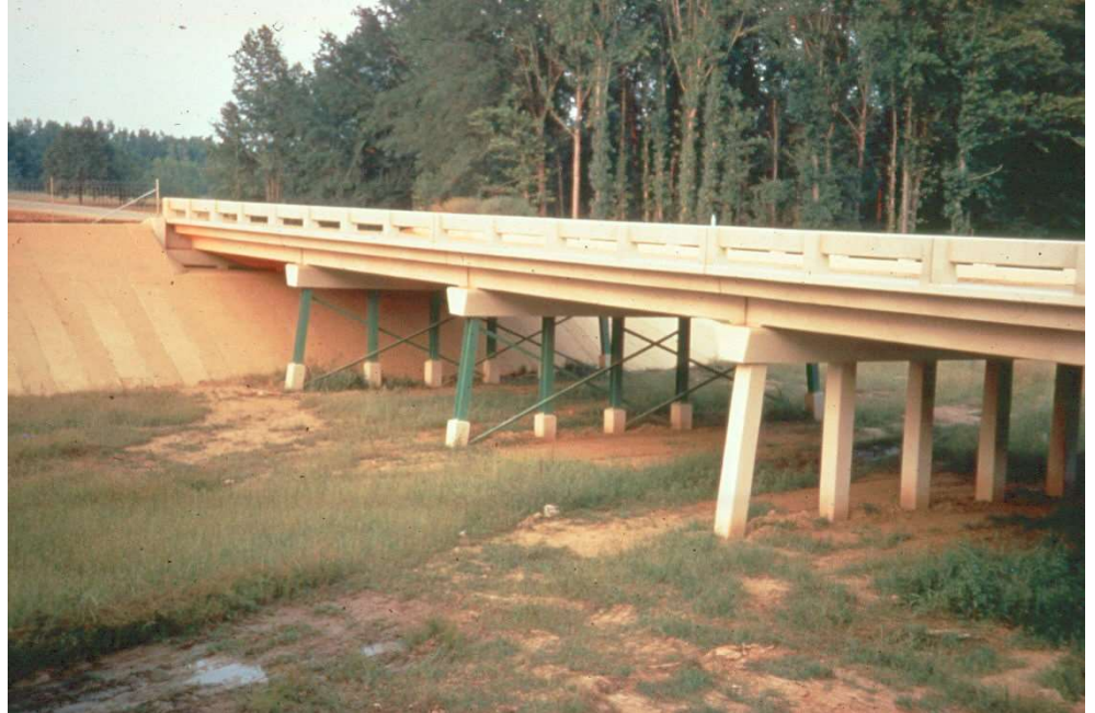
Figure 3.1.81 Pile Bent
