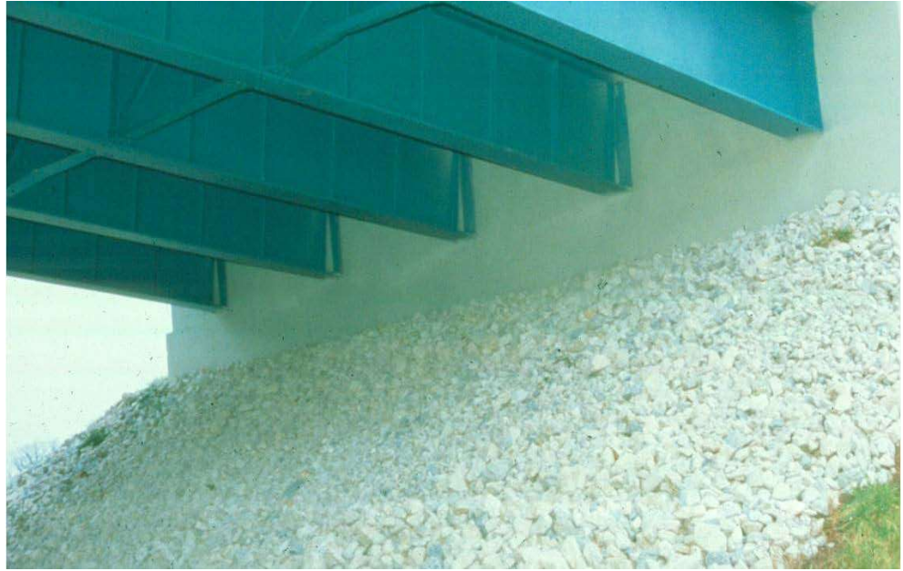
Figure 3.1.74 Integral Abutment
