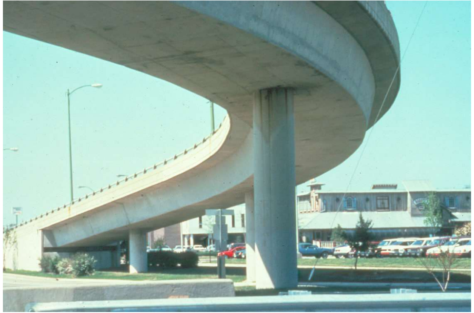
Figure 3.1.77 Column Pier
