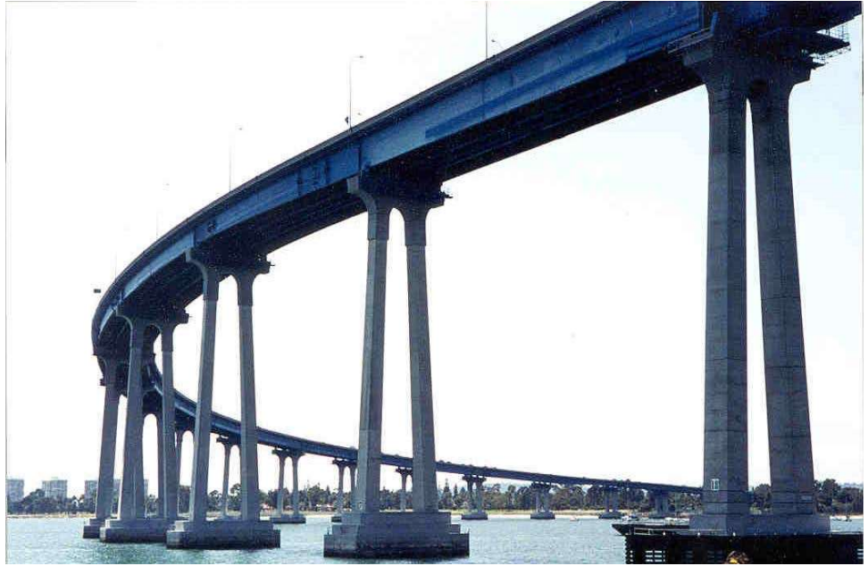
Figure 3.1.48 Curved Girder Bridge
