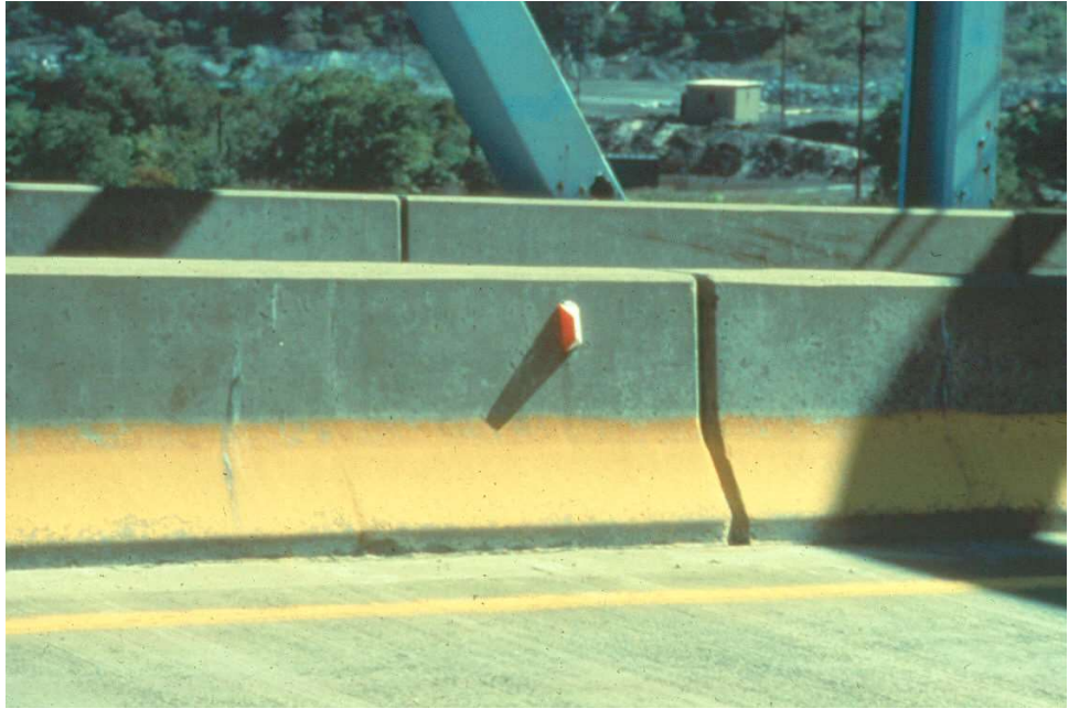
Figure 3.1.40 New Jersey Barrier
