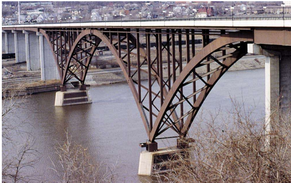
Figure 3.1.64 Main Supporting Members of Deck Arch
