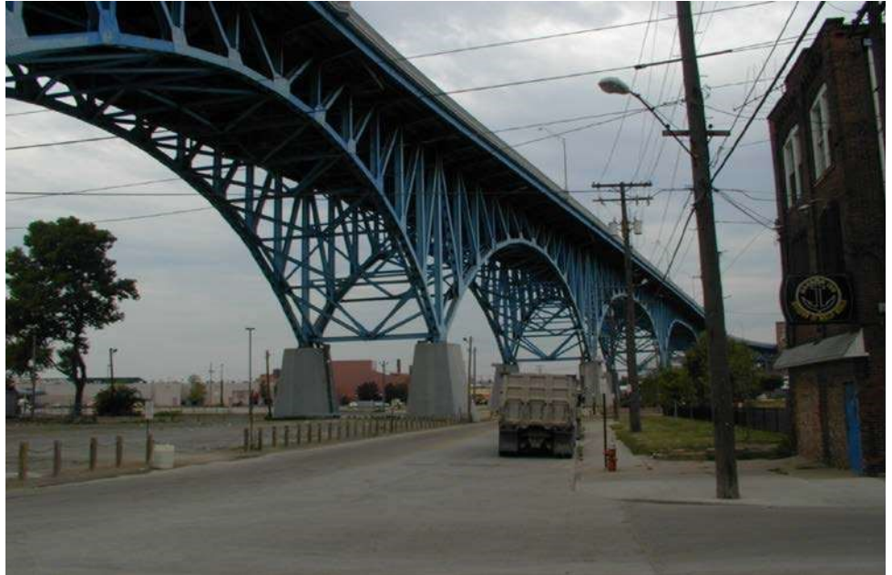
Figure 3.1.52 Deck Truss Bridge
