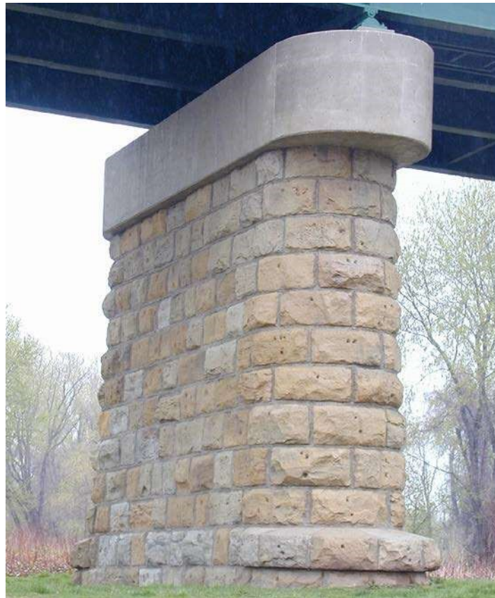
Figure 3.1.76 Solid Shaft Pier
