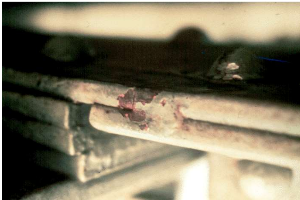
Figure 3.1.25 Close-up of Tack Weld on a Riveted Built-up Truss Member
