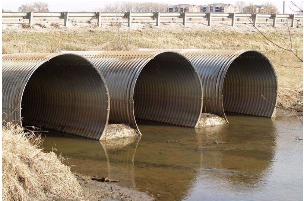
Figure 3.1.84 Flexible Culvert
