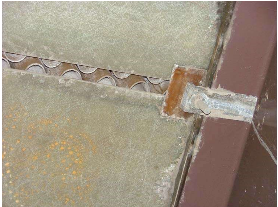
Figure 3.1.35 Fiber Reinforced Polymer (FRP) Deck
