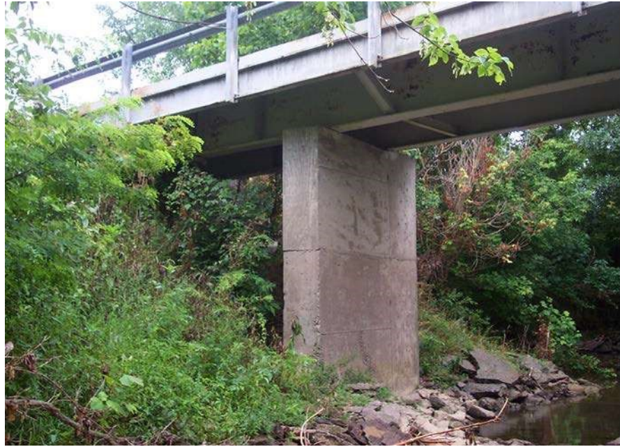
Figure 3.1.75 Solid Shaft Pier
