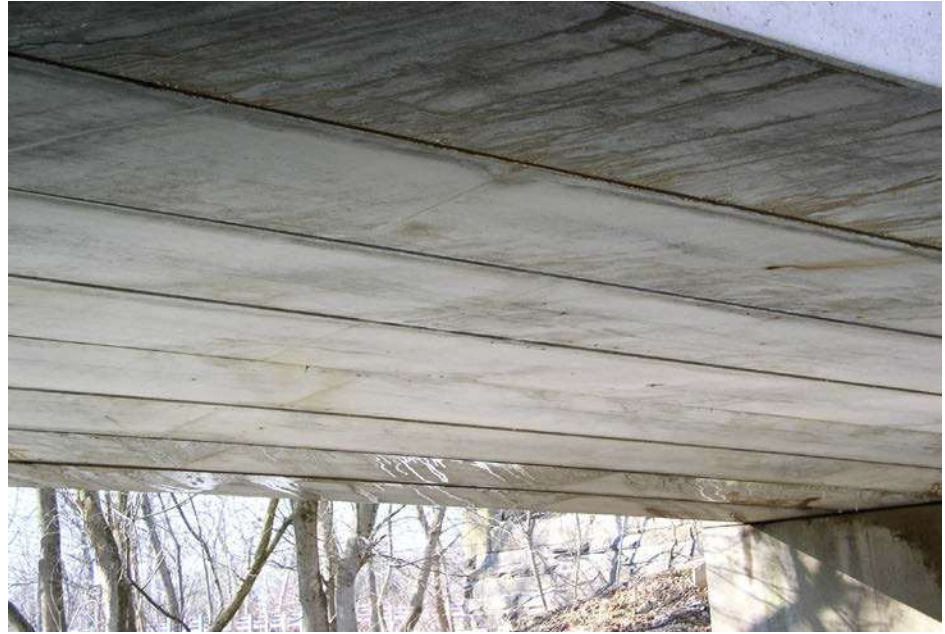
Figure 3.1.50 Adjacent Box Beam Bridge
