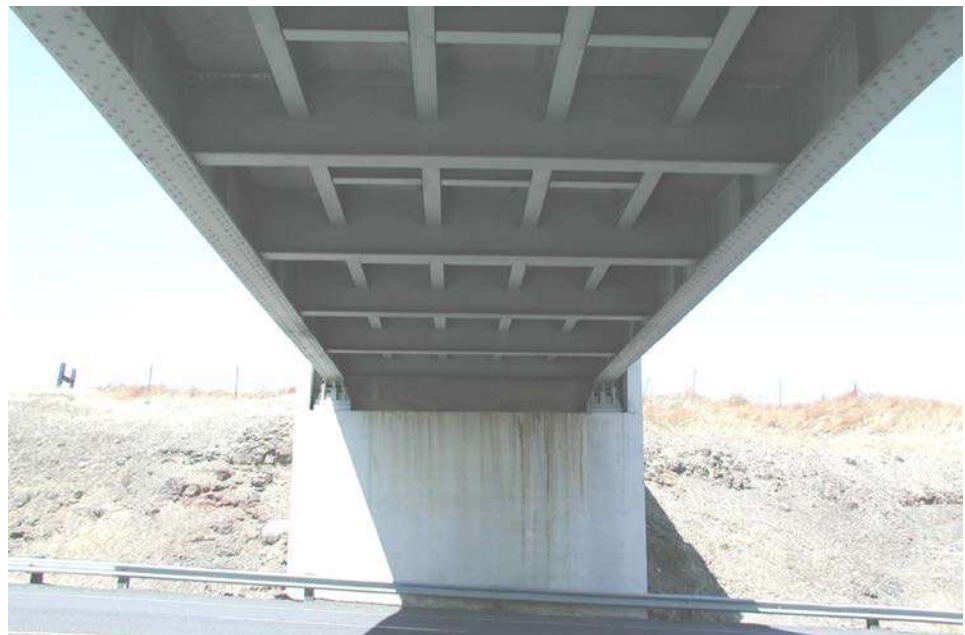
Figure 3.1.47 Girder Floorbeam Stringer Bridge
