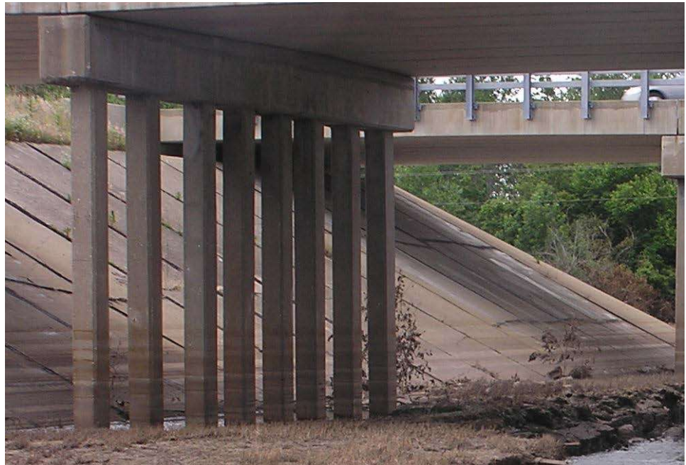
Figure 3.1.10 Concrete Pile Bent
