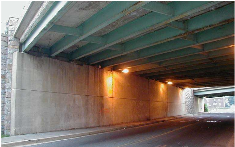
Figure 3.1.71 Cantilever Abutment (or Full Height Abutment)
