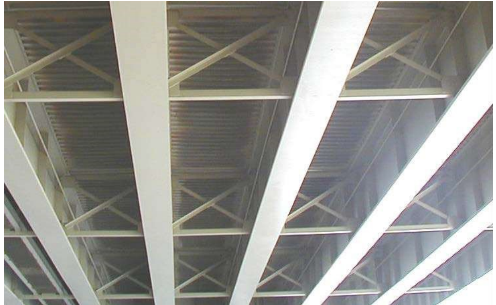
Figure 3.1.66 Cross or X-Bracing
