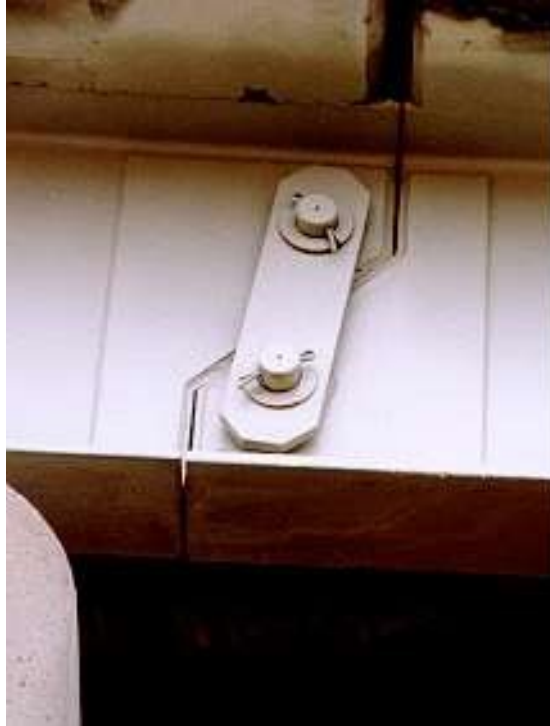
Figure 3.1.26 Pin and Hanger Assembly
