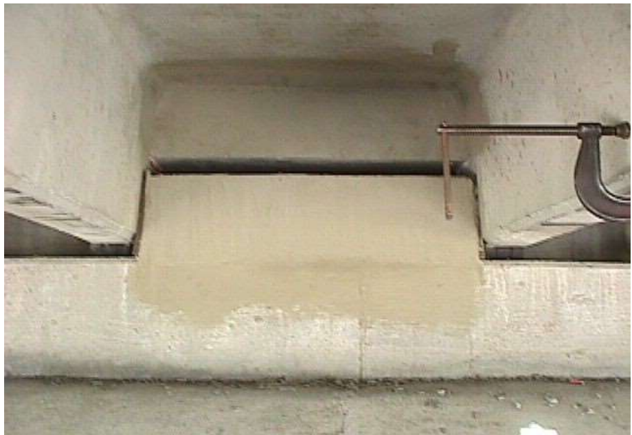
Figure 3.1.49 Tee Beam Bridge
