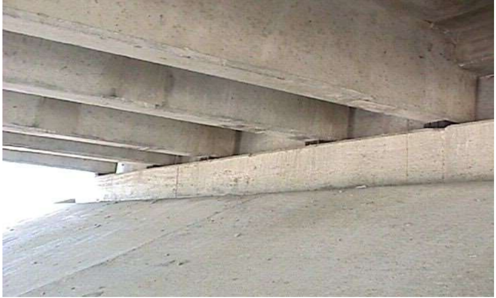
Figure 3.1.72 Stub Abutment
