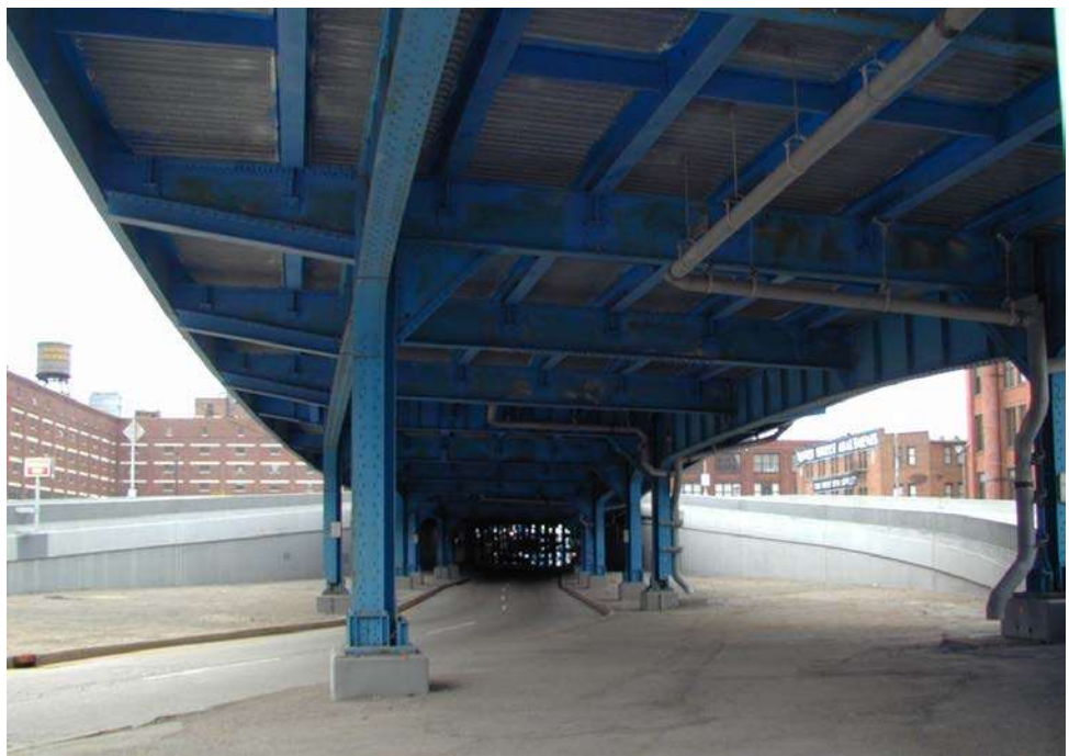
Figure 3.1.80 Column Bent
