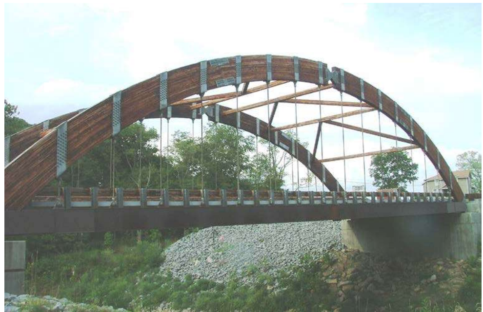
Figure 3.1.55 Through Arch Bridge
