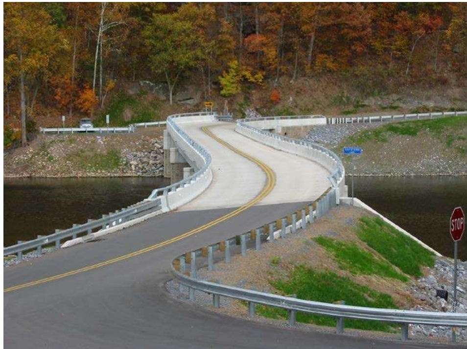
Figure 3.1.28 Bridge Deck with a Smooth Riding Surface
