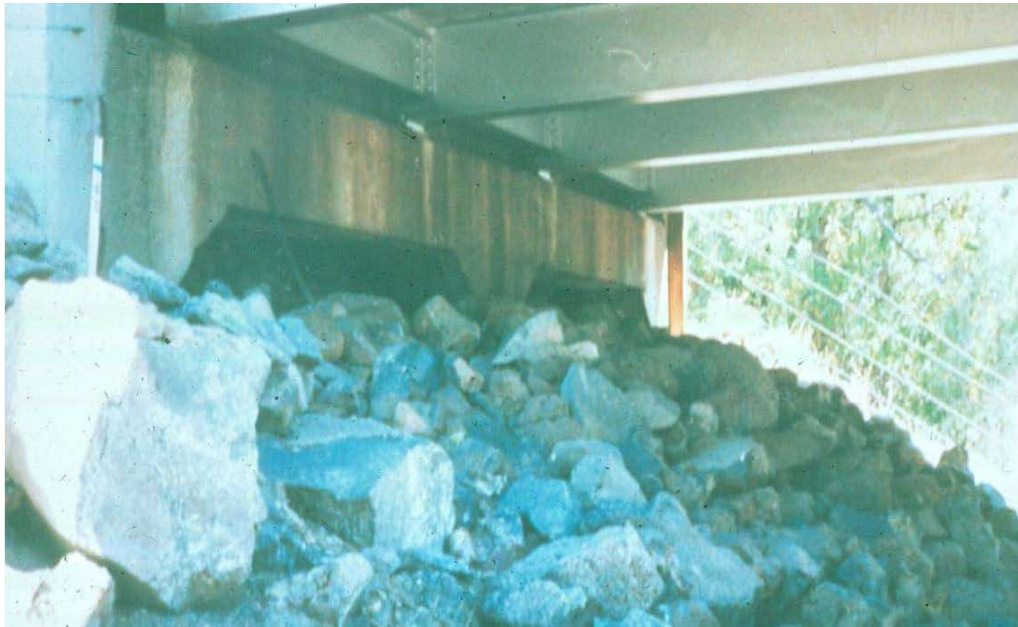
Figure 3.1.73 Spill-Through or Open Abutment
