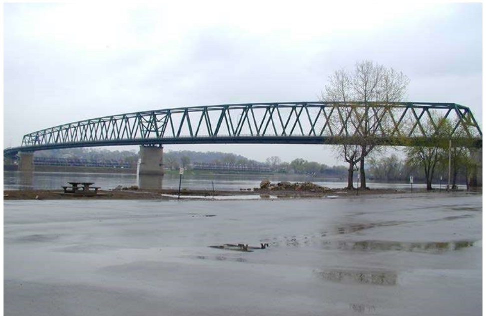
Figure 3.1.53 Through Truss Bridge
