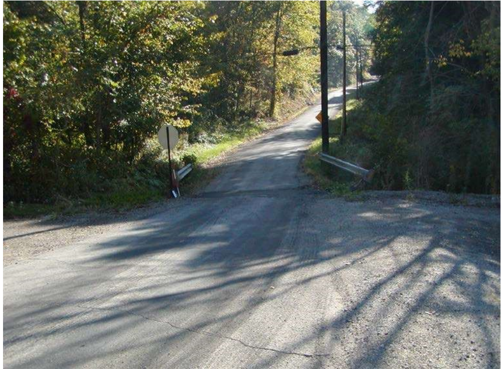
Figure 4.6.1 Near Approach - Toward Bridge
