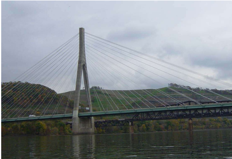
Figure 3.1.20 Cable-Supported Bridge: Cable Stayed
