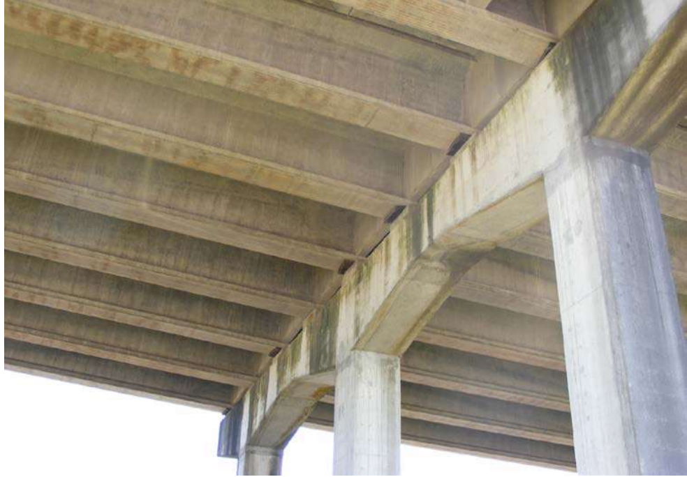
Figure 3.1.46 Multi-Girder Bridge
