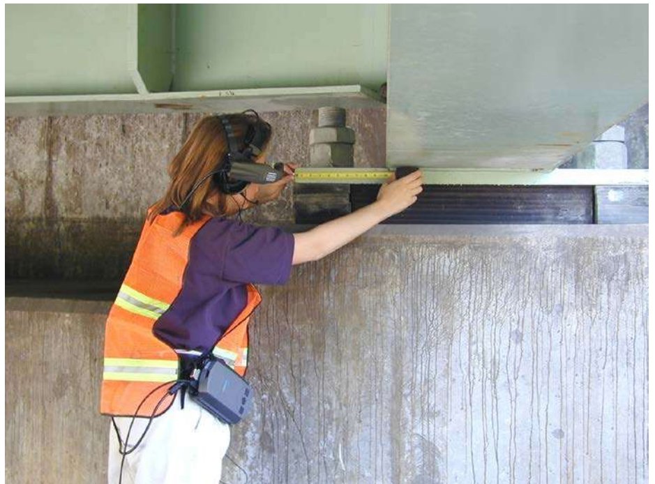
Figure 4.1.9 Inspector Using Wearable Computer
