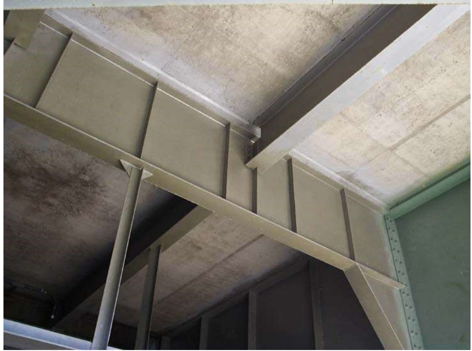
Figure 3.1.29 Underside View of a Bridge Deck
