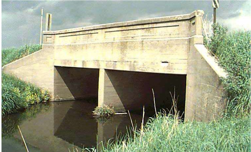
Figure 3.1.83 Rigid Culvert
