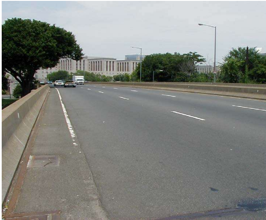
Figure 3.1.36 Asphalt Wearing Surface on a Concrete Deck
